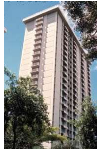
Fig. 2(b). The completed structure with precast façade walls, sunshades, and roof parapets.
