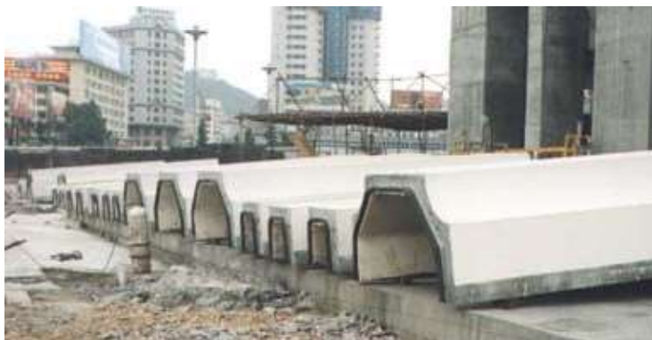
Precast column cladding.
