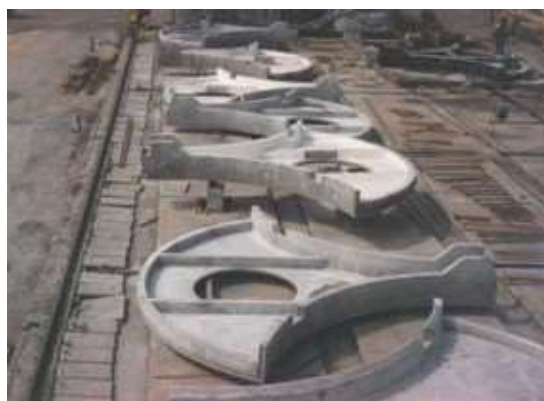
Precast façade panels.
