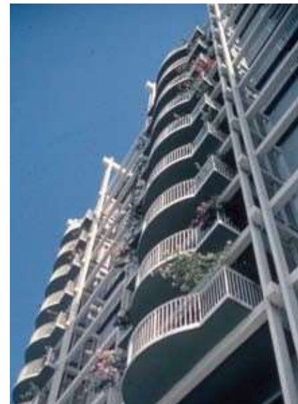
Fig. 1(b). View of the completed latticework and balconies.
