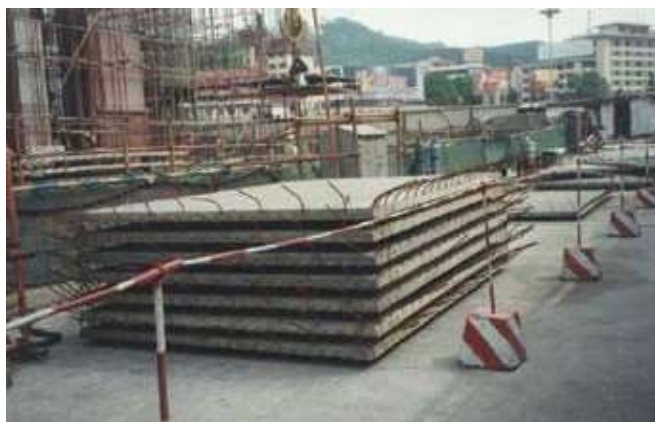
Precast slabs that receive composite cast-in-place topping.
