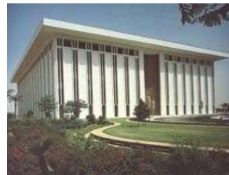
Fig. 4. Headquarters Building, Saudi Arabia Monetary Agency, Riyadh, Saudi Arabia. Precast components include floor beams and slabs, columns, and bearing wall panels.
