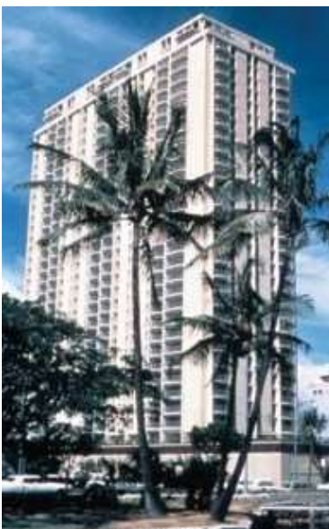
Fig. 3. The 33-story Ala Moana Apartments, Honolulu, built in 1966. Precast components include precast floor slabs with an in situ composite topping, balcony slabs, and wall panels.
