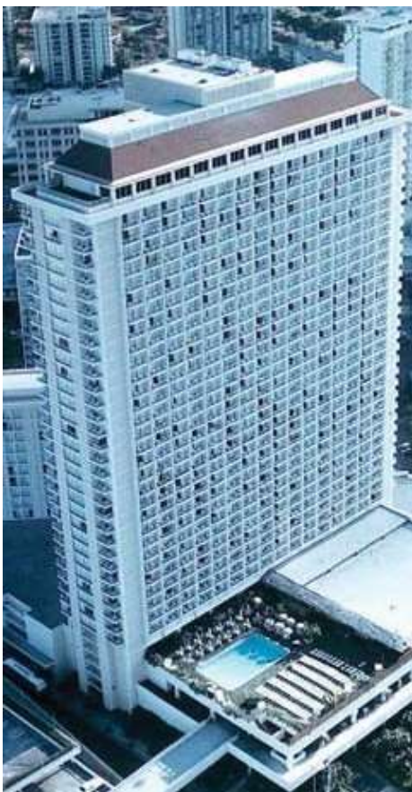
Fig. 17. For the 38-story Ala Moana Hotel in Honolulu, Hawaii, precast column trees were fabricated to support precast floor slabs.
