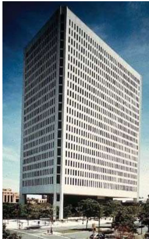
Fig. 16. The 22-story building at 100 Washington Square in Minneapolis, Minnesota. Precast panels were joined horizontally and vertically to form Vierendeel wall trusses.
