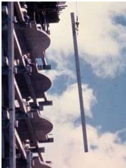
Fig. 1(a). Precast, prestressed trellis beam being erected on the Kahala Mandarin Oriental Hotel in Honolulu, Hawaii.
