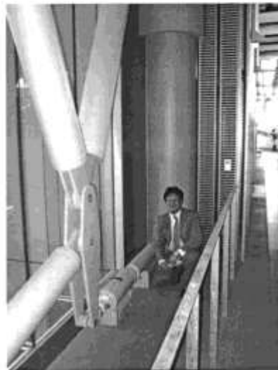
Fig. 17. Nihon-Kagaku-Miraikan, Tokyo National Museum of Emerging Science and Innovation, installed with 30-t MR fluid dampers manufactured by Sawan Tekki Corporation
