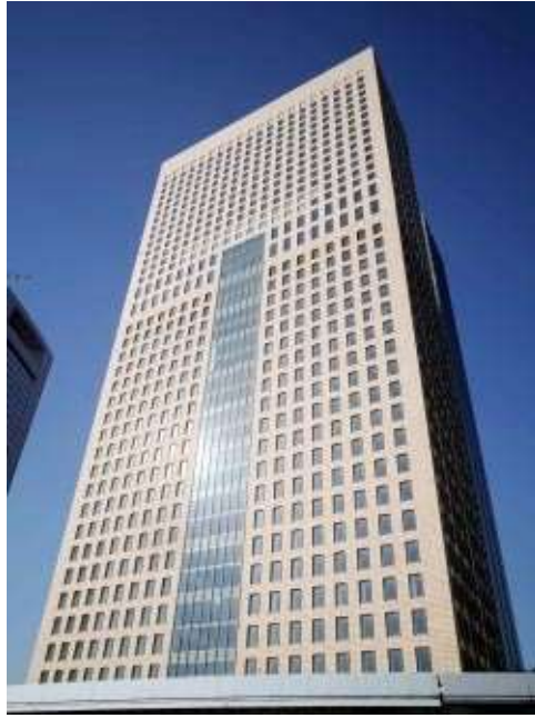
Fig. 15. Siodome Tower under construction in the Siodome area
