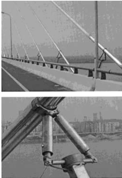
Fig. 18. MR damper installation on the Dongting Lake Bridge, Hunan, China
