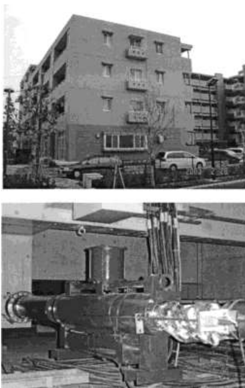
Fig. 20. Base-isolated building installed with 40-t MR fluid damper manufactured by the Sanwa-Tekki Corporation protecting structures against near-source, high-velocity, long-period
