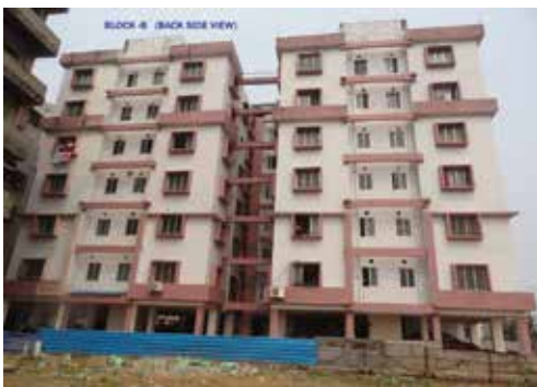
(The Prestige) Block-B Back side view
